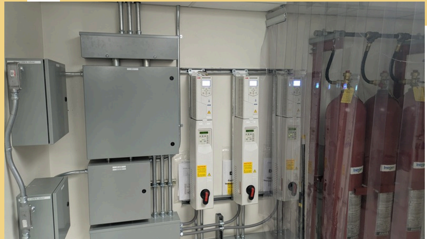
A variety of energy conservation measures were implemented across campus as part of the CECIP program, including variable frequency drives on HVAC equipment and data center hot aisle/cold aisle containment.
